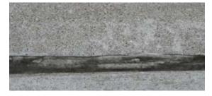
to the crack, pounding it in, then adding caulk, and finally smoothing it out with mineral oil or thinner. However, both sweeping and caulking are time consuming, and caulking may not be realistic for very long or numerous cracks. 6
